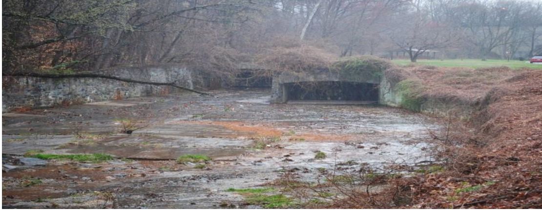
Figure 4. This combined sewer overflow outfall, CSO 49, is the largest in the system. During heavy rainstorms, this spillway can fill up completely due to its massive catchment area of over 2,500 acres. Photo by author, 2014.
