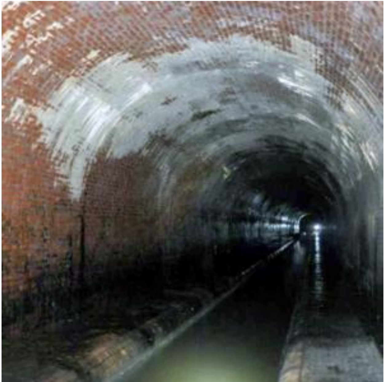
FIGURE 2. INSIDE THE TIBER CREEK COMBINED SEWER, JANUARY 2017. THIS TYPE OF SEWER FEATURES A CENTER CHANNEL OR CUNETTE THAT IS OVERARCHED BY MULTIPLE COURSES OF BRICK DURING HEAVY RAINS, THIS ENTIRE TUNNEL WILL FILL WITH COMBINED SEWAGE.
